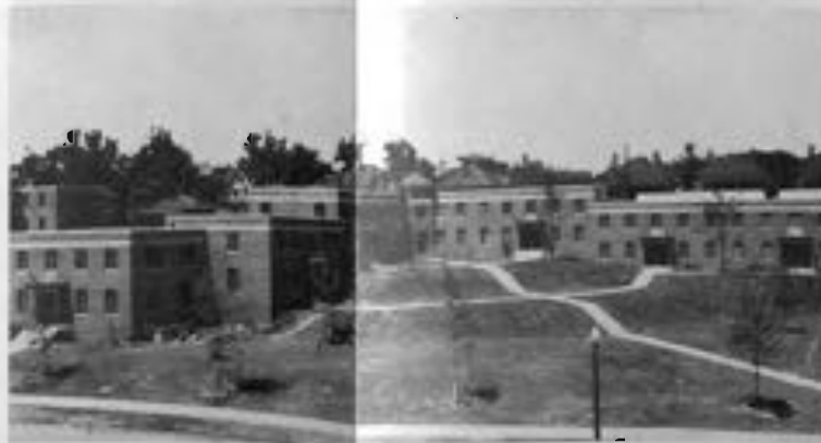
TECHWOOD HOMES, ATLANTA, GA. Before and After Views
